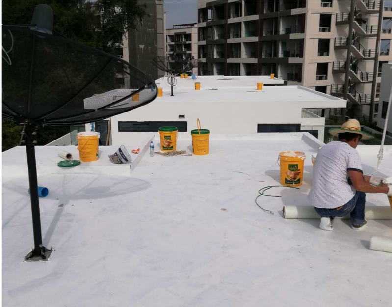
Locates in Pattaya, with acrylic waterproofing coating.
